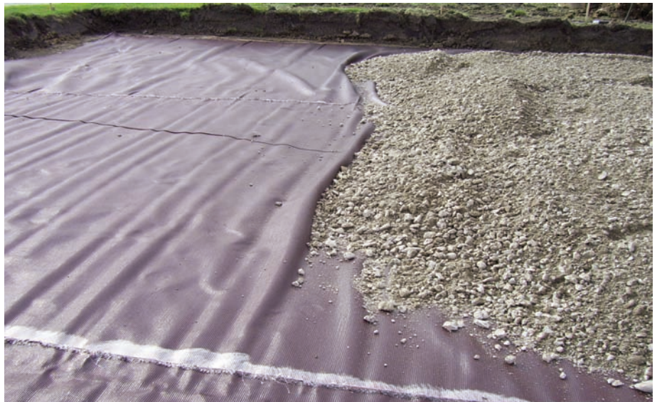
Glued seams allow RS380i to stay in place and maintain overlap while being installed
