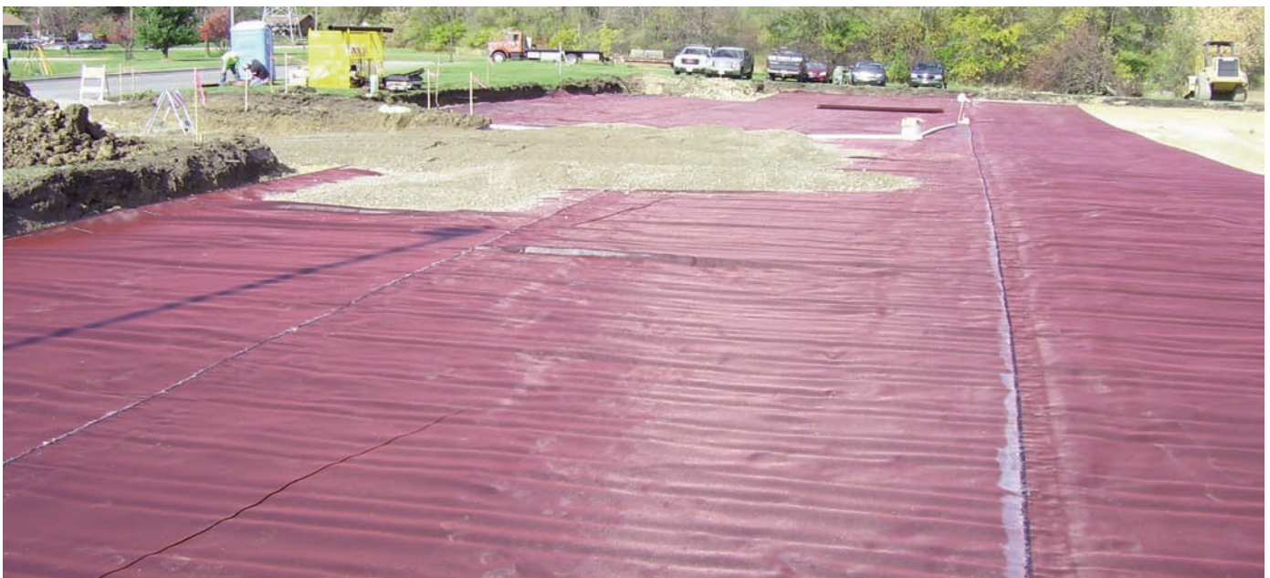
Stone being placed over Mirafi® RS380i.
