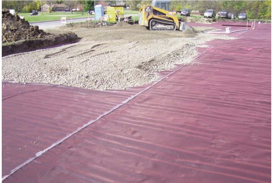
Stone continues to be placed using lightweight equipment
