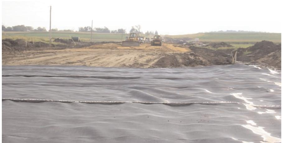
Due to the soft, peat subsurface, Mirafi® HP770PET was required to complete the road widening project
