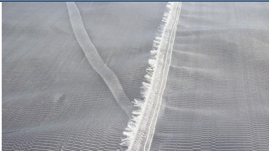
A prayer seam was used to stitch the panels of Mirafi® HP770PET.
