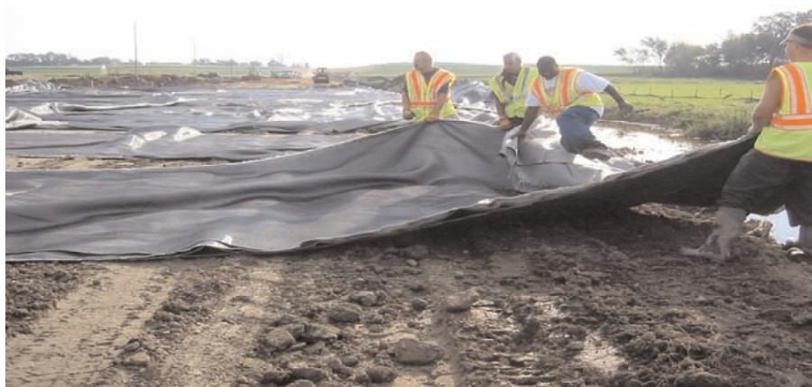
After the Mirafi® HP770PET panels were seamed together, 3m (10ft) of fill soil was installed and left for 4 months to compact the excess pore pressure of the peat.
