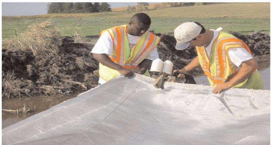
Overlapping the fabric would allow the mud to move up between the panels. Seaming was required to maintain 100% coverage.
