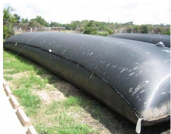
Figure 1. 30'circumference x 50' long Geotube® unit in sand drying bed effectivly increases the capacity of the drying bed to dewater more sludge.
