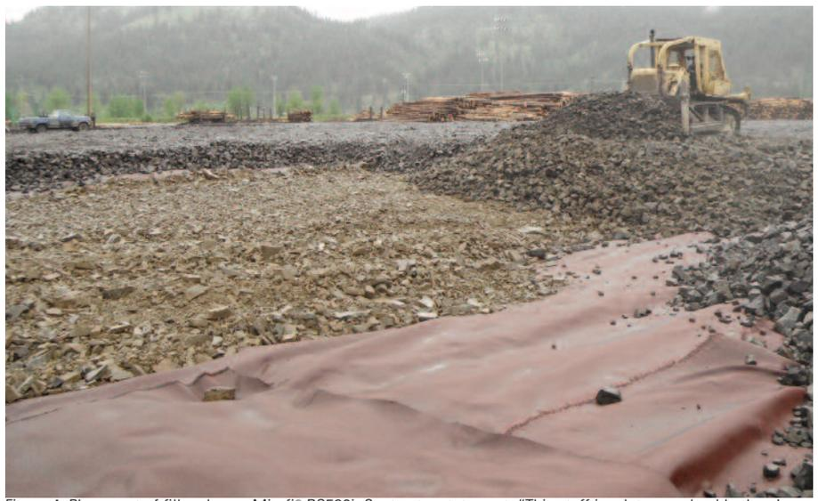
Figure 4: Placement of fill rock over Mirafi® RS580i. Contractor statement: "This stuff is a lot more durable than I thought."
