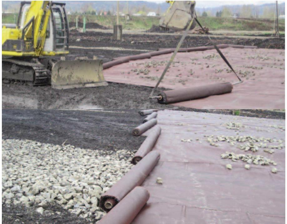
Figure 3: Installation of Mirafi® RS580i using a track-hoe with 1-3 feet of overlap.
