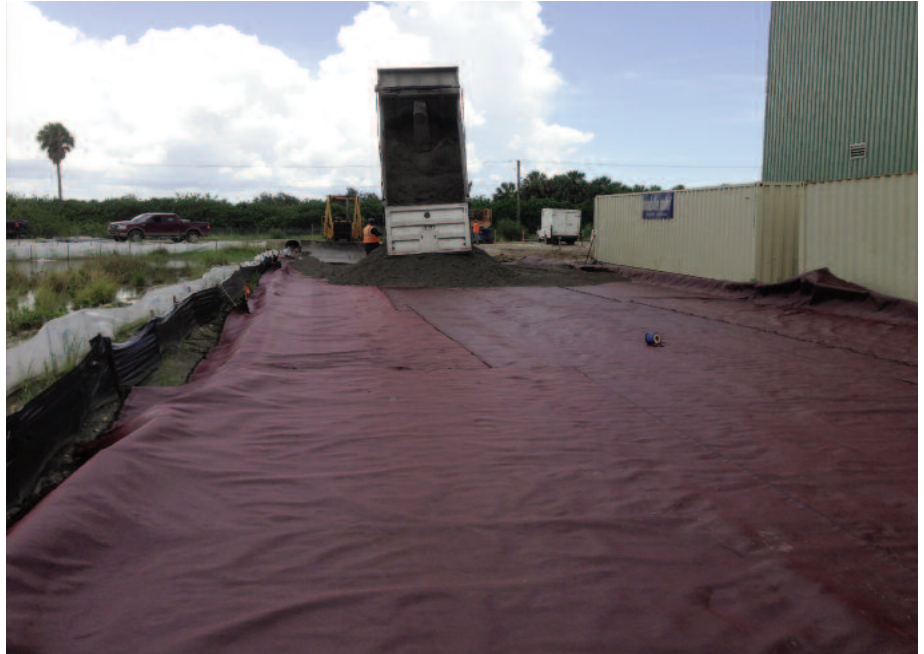
Placing lift of Limerock Base aggregate over panels of Mirafi® RS580i.
