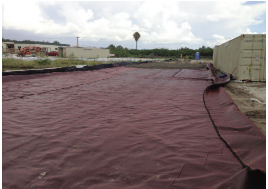
Placed panels of Mirafi® RS580i geotextiles.
