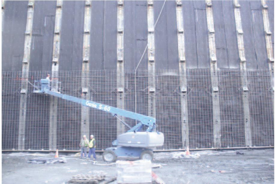
Placement of rebar mat to receive shotcrete.
