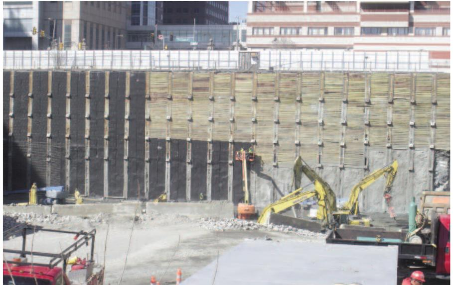
Placing Mirafi® G-Series drainage composite against lagging.
