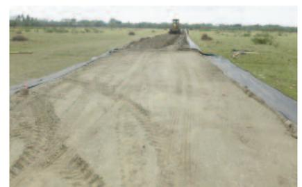
Installation of subbase on top of Mirafi® HP570.
