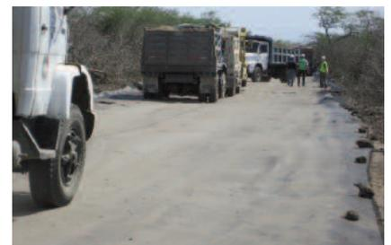
Multiple trucks hauling stone to the site on Mirafi® HP570 without damage.
