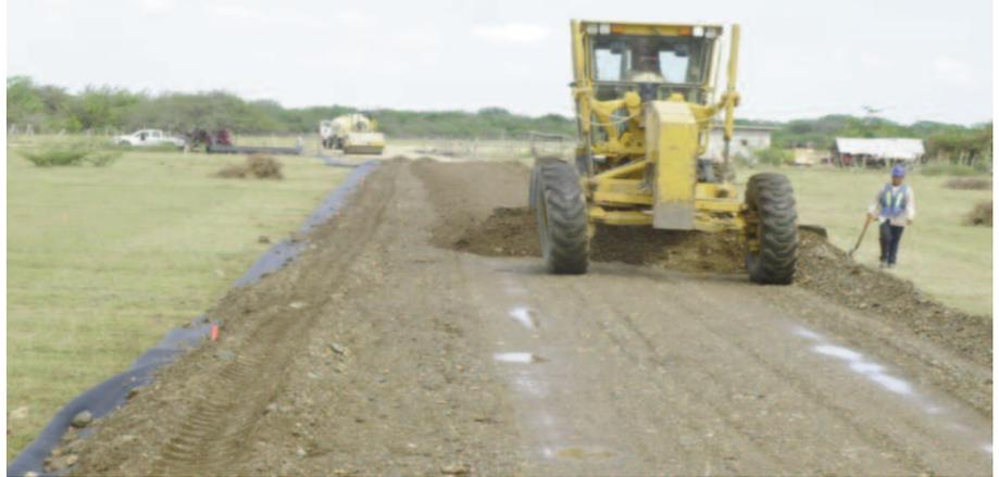
Water being added to the subbase over Mirafi® HP570 for proper compaction.
