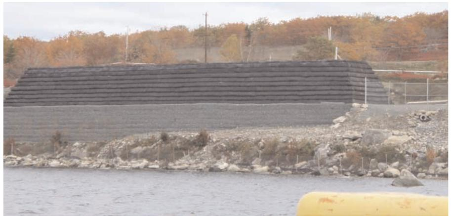
Complete 6.0m (20ft) blast wall situated on top of a 6m (20ft) MSE structure.
