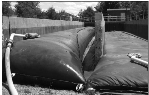
Two 100ft long Geotube containers were placed in the sedimentation basins.
