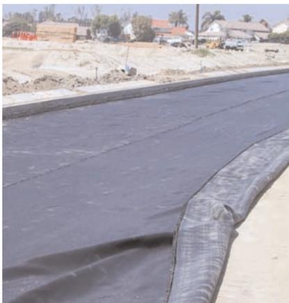
Mirafi<sup>®</sup> HP570 was selected for this project because of its high modulus at low strain and high tensile characteristics.
