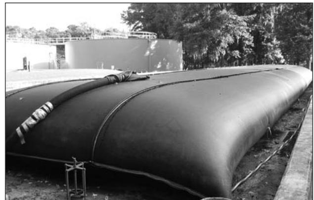
Water Oak Utility saved over \$33,000 dewatering with Geotube® versus liquid hauling and dewatering on the first Geotube® installed.
