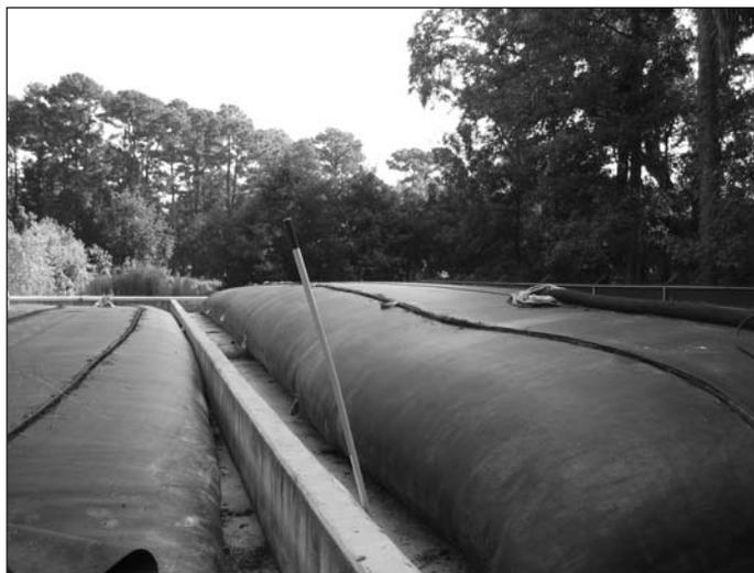
730,000 gallons of sludge at 2% solids have been dewatered in Geotube® #5 which is still in use.
