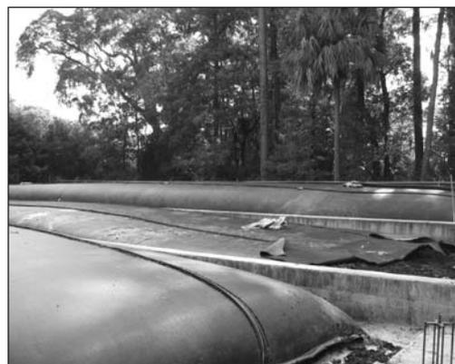
Five Geotube® containers were installed in series to allow one to be removed while four were in operation.
