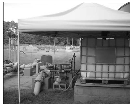
Proper polymer mixing and injection helps to provide good chemical conditioning.
