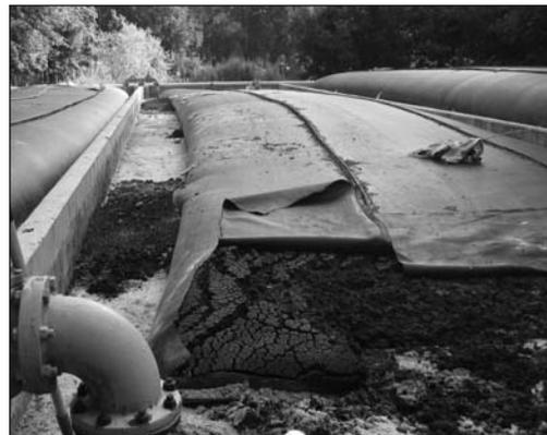
In 19 months, over 3,000,000 gallons of sludge have been dewatered with Geotube® technology.
