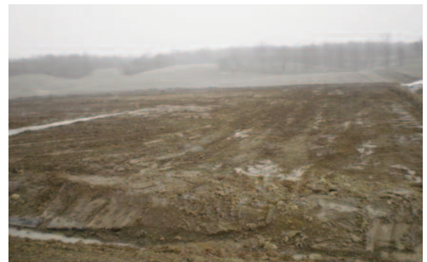
Preparing the grade.
