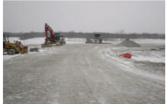
Mirafi® HP570 kept the project on schedule - regardless of weather.
