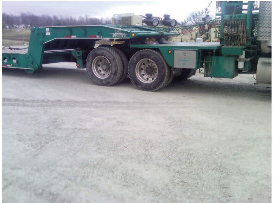
Finished drive area. No rutting under the loaded semi trucks.
