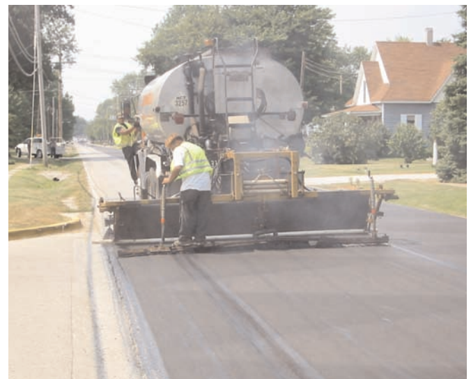
Mirafi® MPV500 can increase the chip seal service life by 60%.
