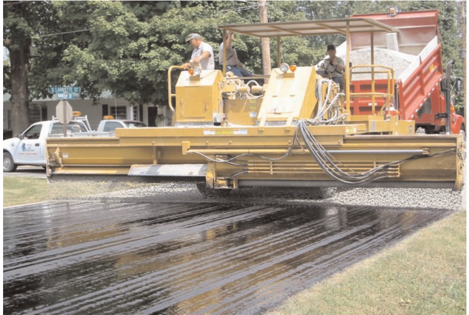
Above: The chip seal aggregate was applied using a variable width spreader.
