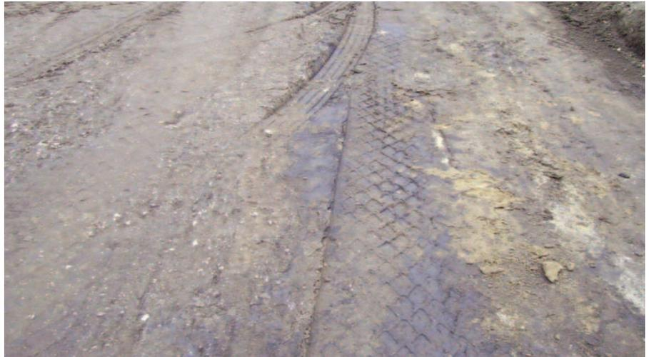
The existing high-moisture soil subgrade was unable to pass the proof roll.
