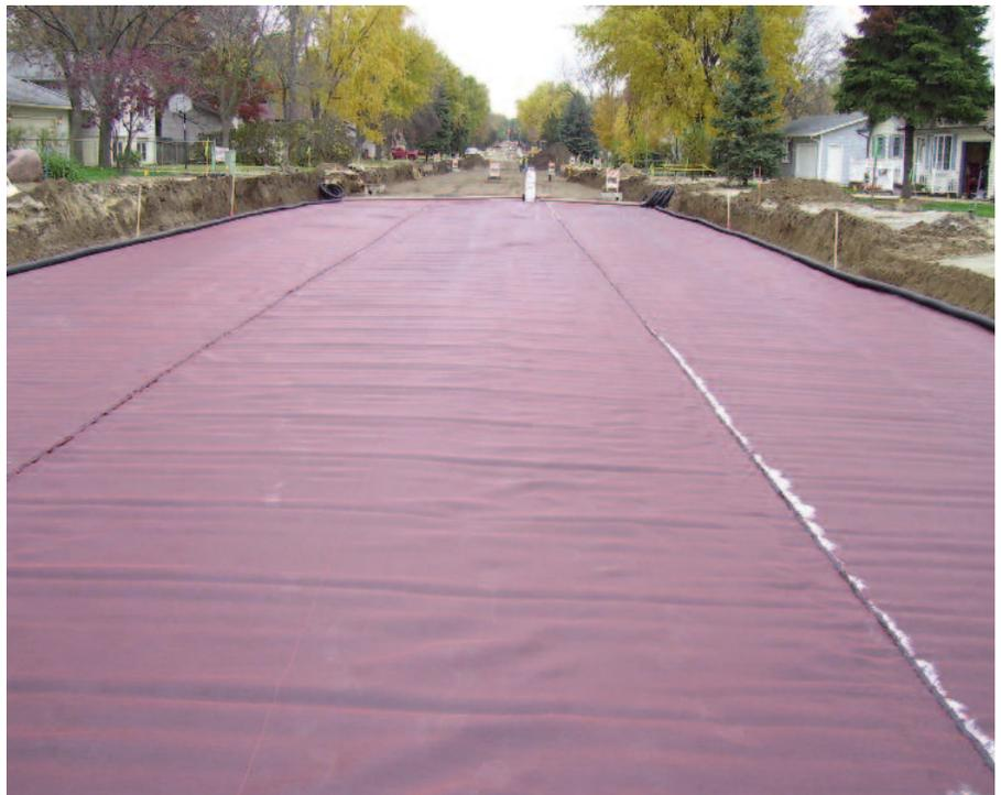
Mirafi RS380i lays flat and goes into tension well. Maintaining overlap was no problem using 3M Geotextile Seaming Cylinder Spray Adhesive.
