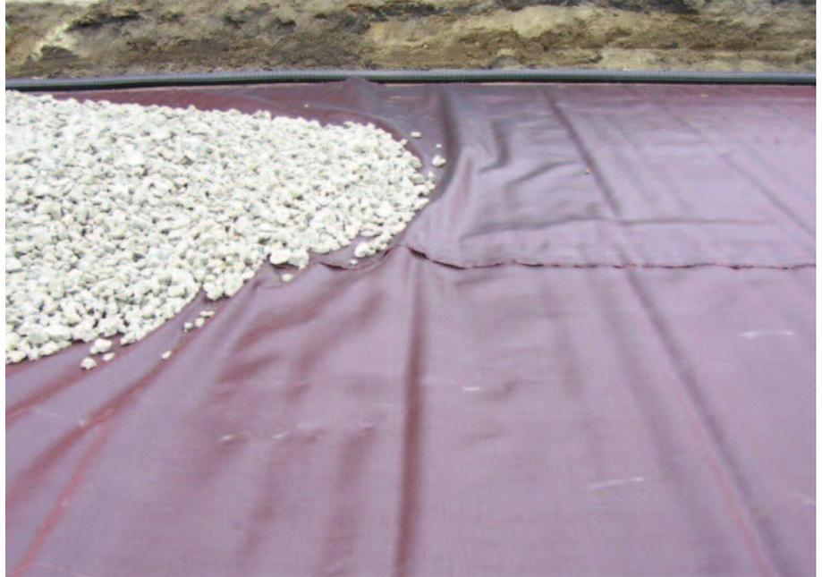
Wrinkles are easily pushed in front of the geotextile when pushing aggregate from one end and the orange color let the equipment operator know right where it was.
