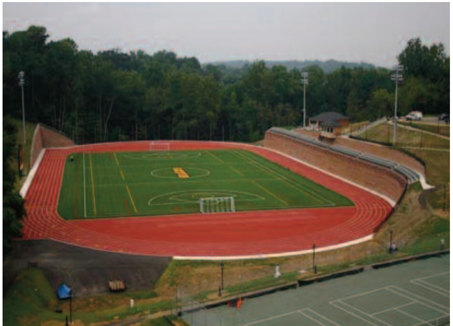
Randolph College completed athletic facility.
