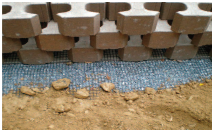
Backfill brought up and compacted prior to placement of drainage aggregate.
