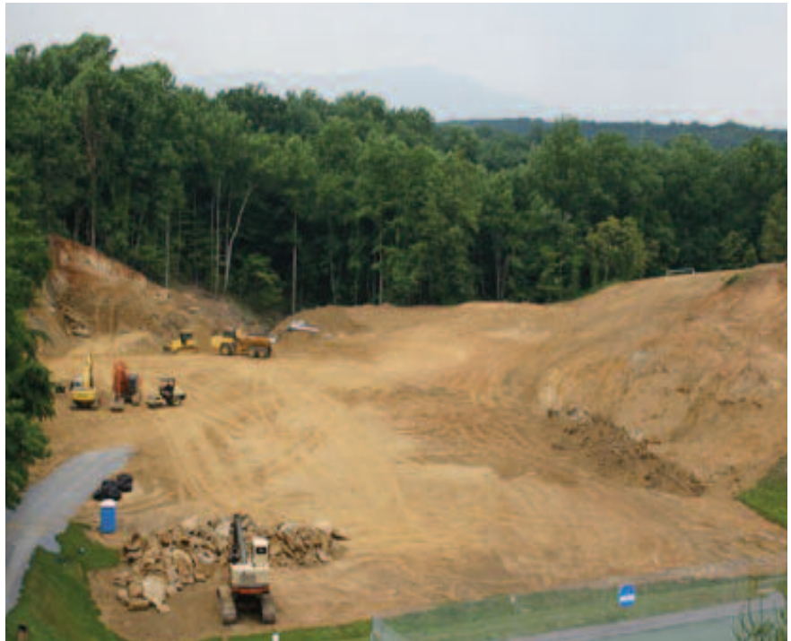
Site prior to retaining wall construction.
