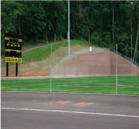
Retaining wall was needed to stabilize the cut slope.
