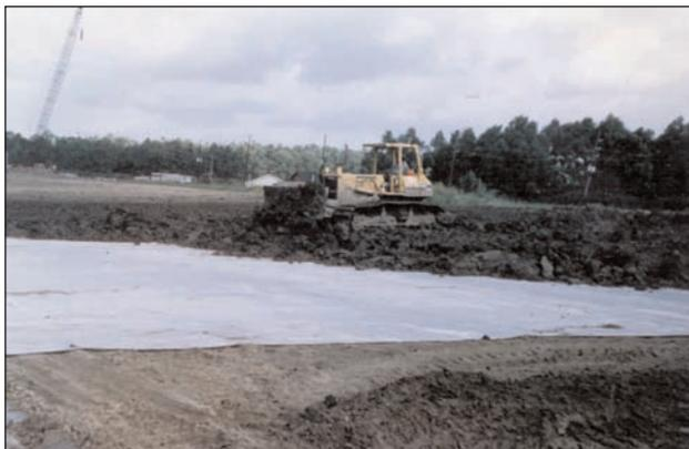
Though both the geogrid and geotextiles performed as expected, the geotextile is the logical choice for this application.
