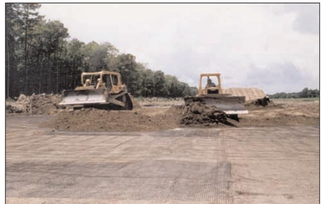
The installed cost of the geogrid test section was 46% more than the installation cost of the Geolon® geotextile.
