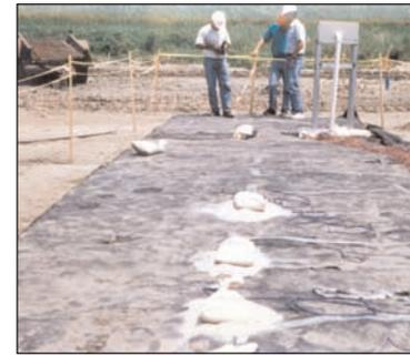
Monitoring instrumentation was placed within the levee.
