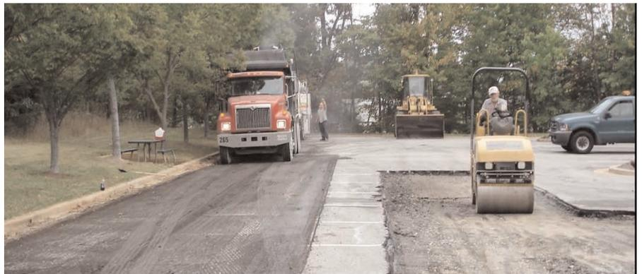
Recompaction of base course in test pit areas and edge milling being preformed.
