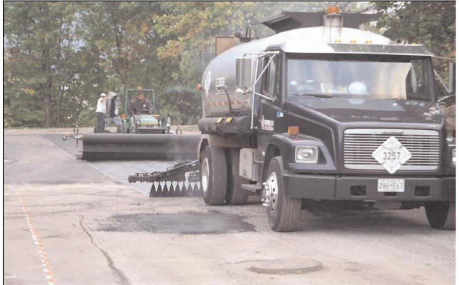
Distribution truck shooting PG64/22 asphalt cement with paving fabric being placed behind it.
