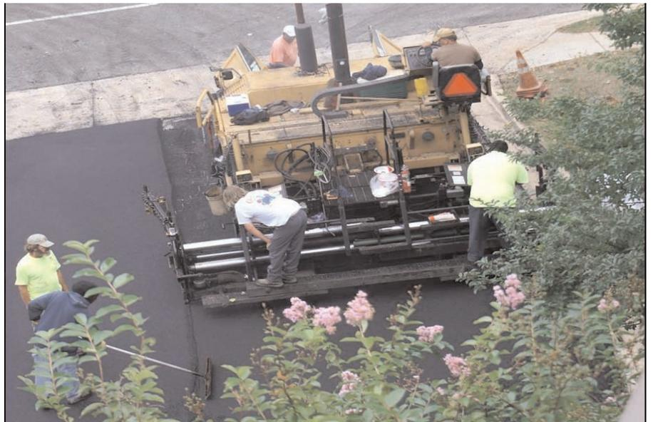
Asphalt surface mix being placed.
