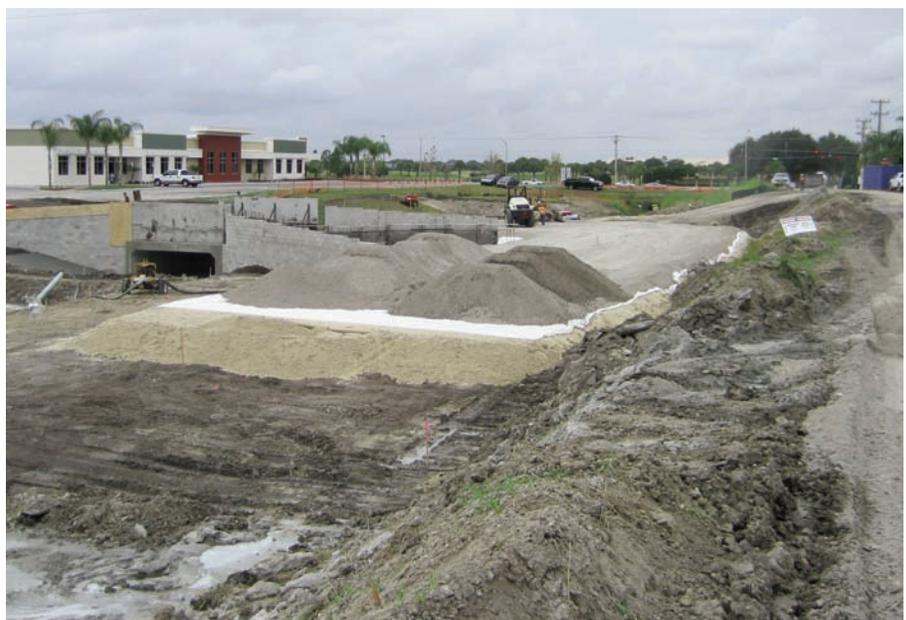
Installation of structural fill over Mirafi® HS400.
