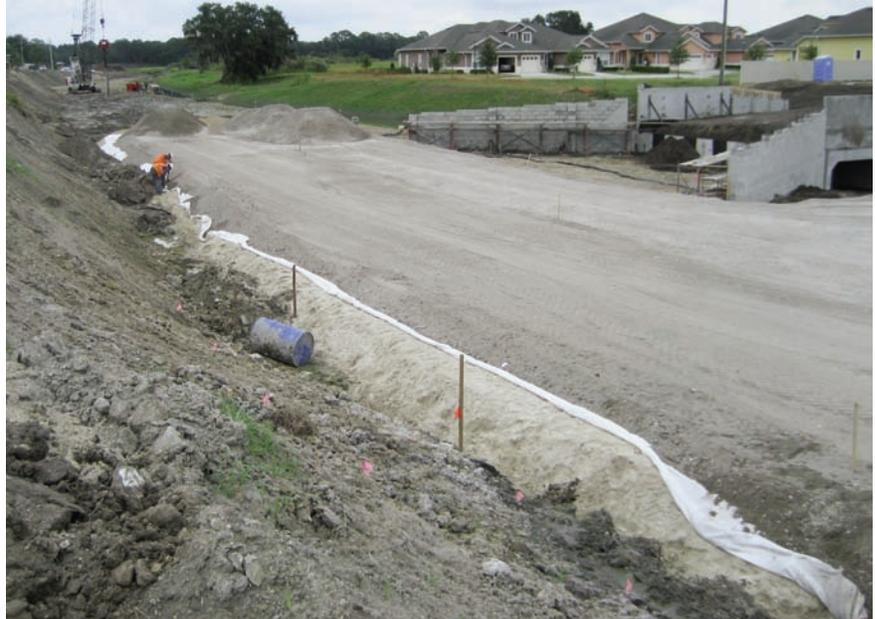
Installation of the structural fill on top of Mirafi® HS400 .
