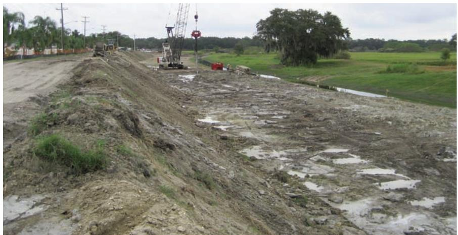
Installation of Cast-In-Place piles prior to the geosynthetic installation, showing pile caps.
