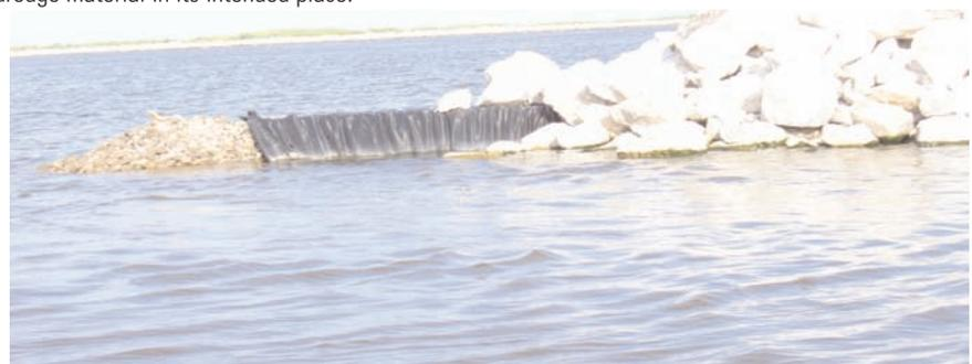
1x4 aggregate and 2,200 lb. rip rap with Mirafi® FW404 used as a separation geotextile
