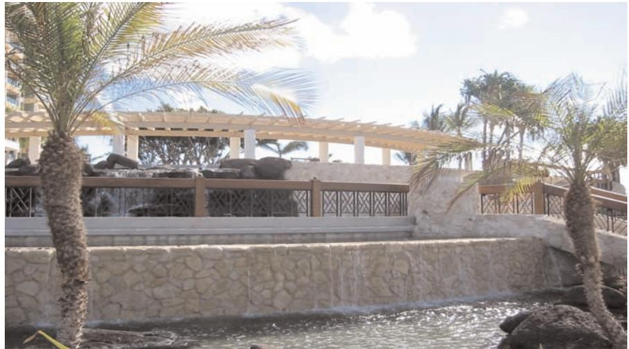
The completed 13.5ft Mirafi® HS400PP wrapped wall supports the shotcrete facade.
