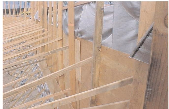
Wooden forms create the vertical face. Mirafi® HS400PP was placed up the back of the form.
