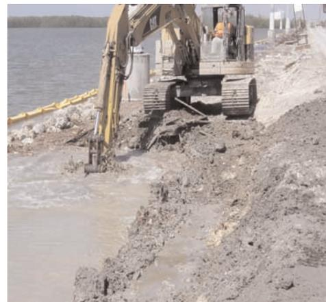
Trench dredging for platform of temporary retaining wall.
