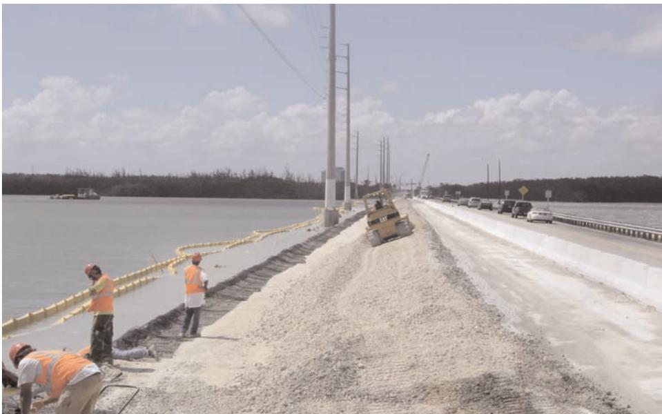
Gravel in-fill within temporary retaining wall along US 1.
