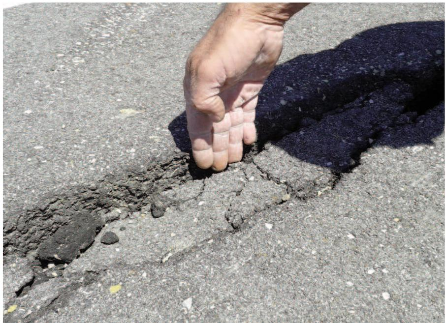
Depth and width of cracking on Highway 106 made for very poor rideability and dangerous conditions.
