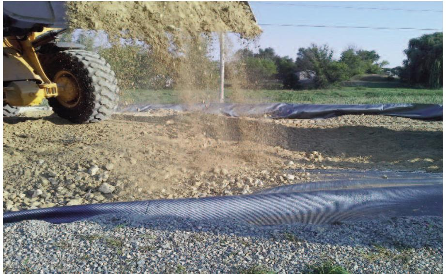
Loader adding first lift of aggregate on Mirafi® H<sub>2</sub>Ri.
