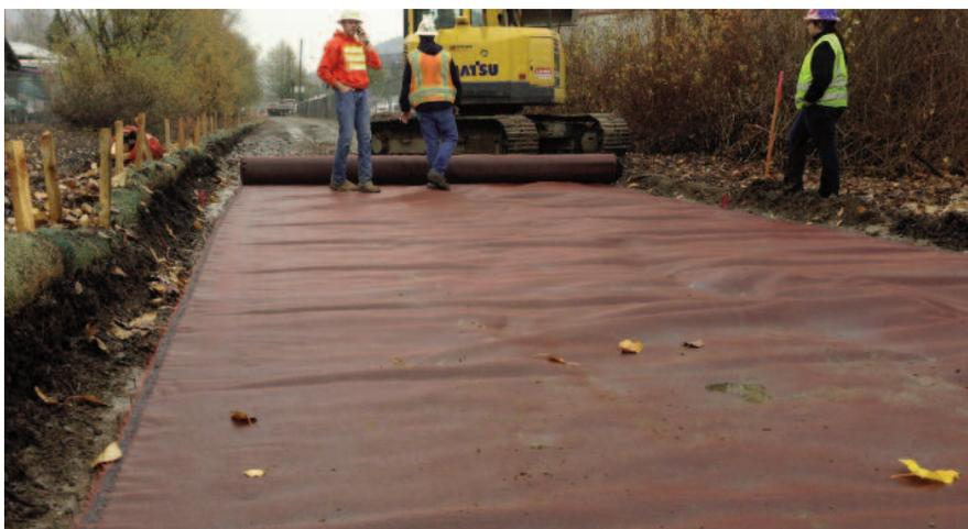
Installation of Mirafi® RS580i over the soft subgrade was done with ease thanks to the 17' wide rolls and strength of the product.
