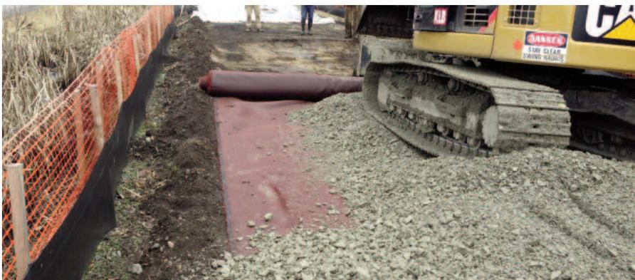
Mirafi® RS580i provided immediate support over the saturated subgrade for equipment loading.
