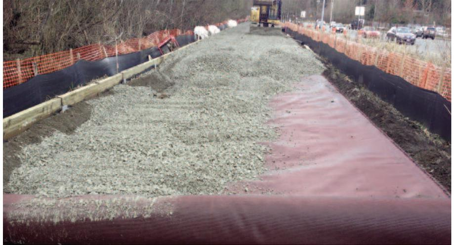
Mirafi® RS580i demonstrating immediate aggregate interaction (interlock) over a soft subgrade.
