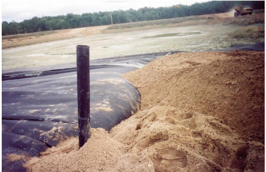
When ground displacement did occur, the geotextile stretched with the deformation of the sludge in a tensioned membrane effect.
