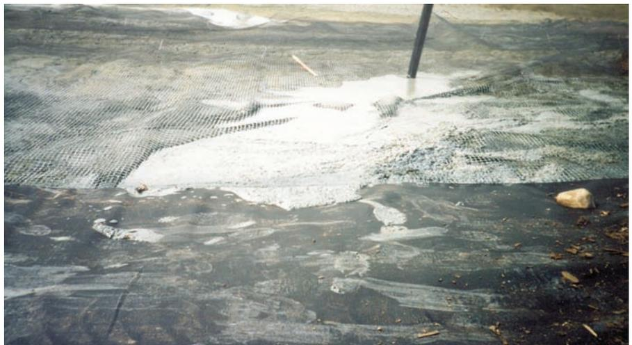
Mirafi® HP665 prevented sludge from flowing up through the geotextile, the geogrid did allow the contaminated mud to soak through into the overlaying fill.
