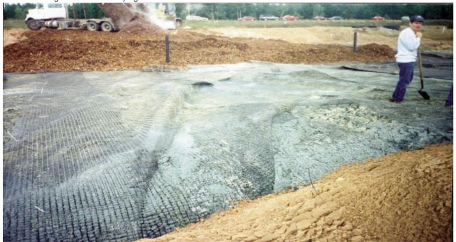
When ground displacement did occur, the geogrid stretched with the deformation of the sludge and split apart.
