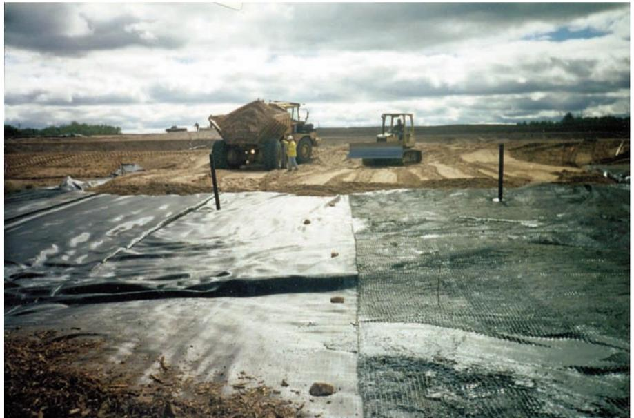
The Mirafi® HP665 provides for uniform load distribution, prevents movement of the contaminated sludge into the granular fill, and has more appropriate strain for this sludge cap than the geogrid. The geogrid could not stop mud flow.
