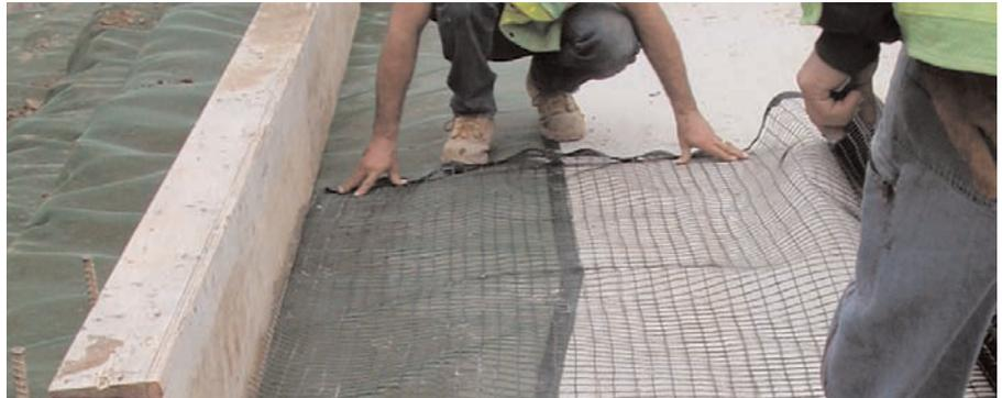
**Above:** Overlap required between primary reinforcement and face wrap.
