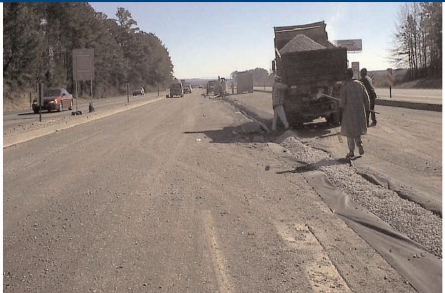
Filter fabrics used in trench applications prevent clogging and decreases aggregate settlement.
