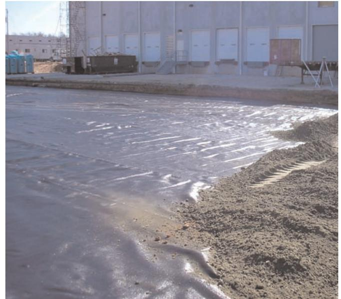
Starting placement of Mirafi® HP570 and base course under asphalt pavement adjacent to the concrete truck dock area.
