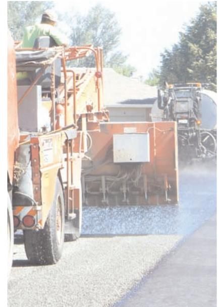
Installation of the CRS-2 and 3/8" chips over Mirafi® MPV500 on 35th St. Ct.
