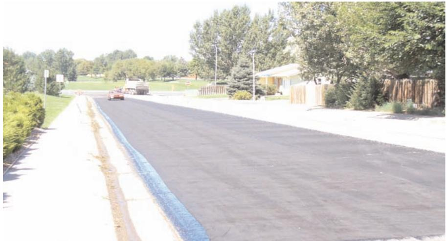
9th Street during installation. Paving fabric is on left and under the chip seal on the right.
