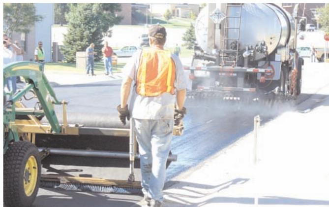
Installation of the PG64-22 and Mirafi® MPV500 on 35th St Ct.
