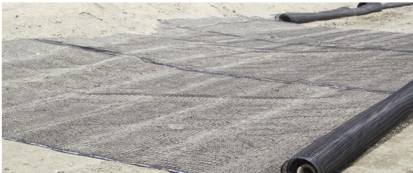
Multiple layers of Miragrid® 8XT placed across the entire embankment width.
