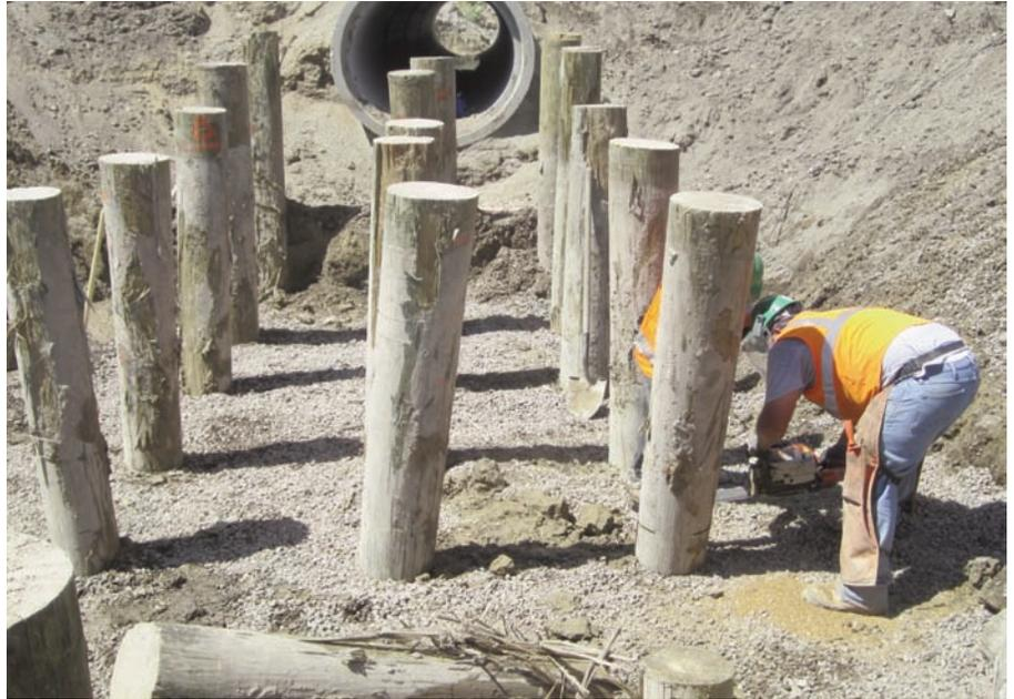
Timber piles being cut to design lengths.
