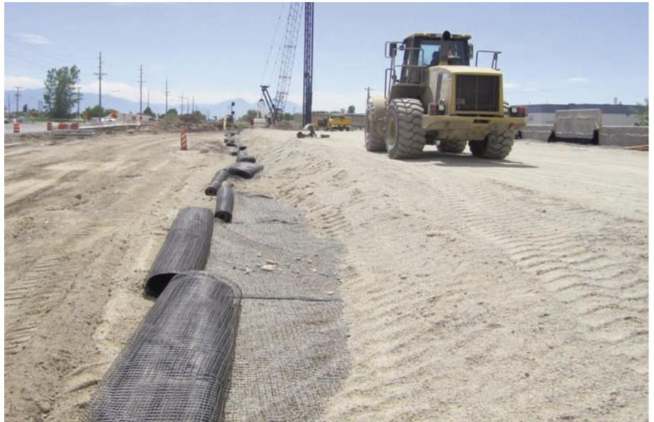
Two foot thick compacted stone and sand backfill between the Miragrid® 8XT layers.
