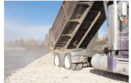
An end-dump is used to place the rock onto the geotextile.
