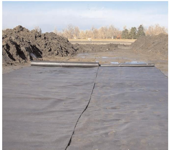
Mirafi® HP570 installed with appropriate overlap.
