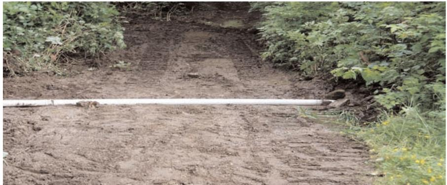
Low lying muddy area that floods during the winter months. Contractor placed a 6 inch PVD drainage pipe to allow free water flow underneath the subgrade
