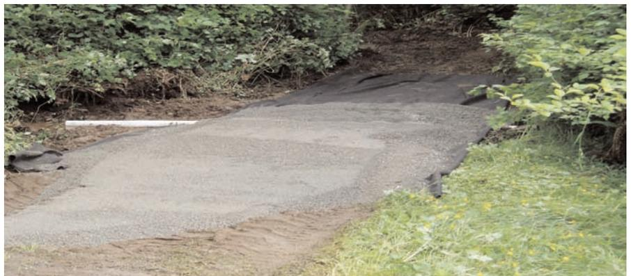
Placement of 5/8" crushed rock over the Mirafi® 160N geotextile
