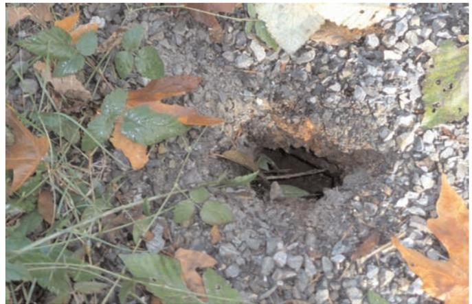
Burrowing rodents like moles; create unique dangers for riding horses on the trails. Mirafi® 160N was used to bridge this hole and prevent rodents from trying to burrow to the surface again.
