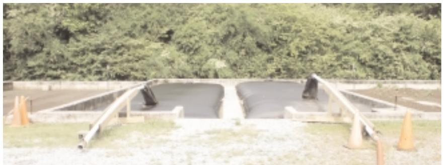
Geotube® containers being filled with solid waste pumped from the digester. Two tubes fit within this drying bed. The city of Eatonton is pleased with the Geotube® Containers.
