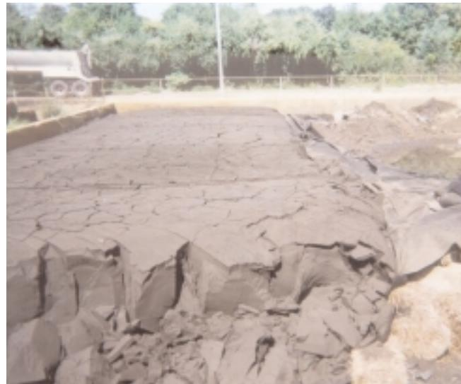
**Step 4: Removing Dewatered Solids**
