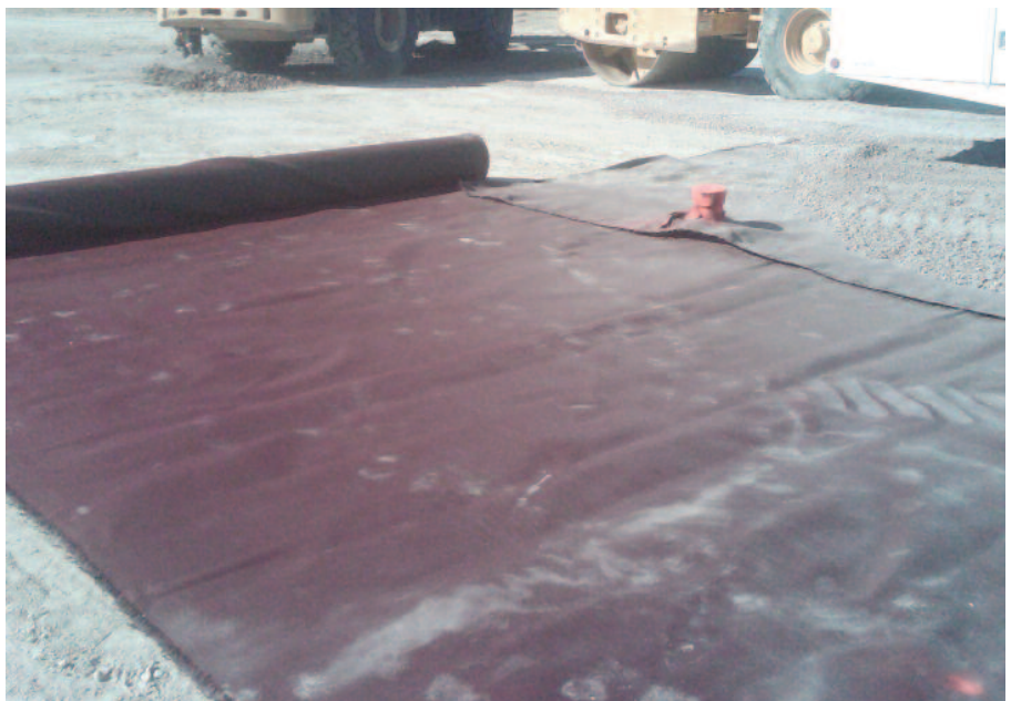
Mirafi® RS580i rolled out and overlapped appropriately.
