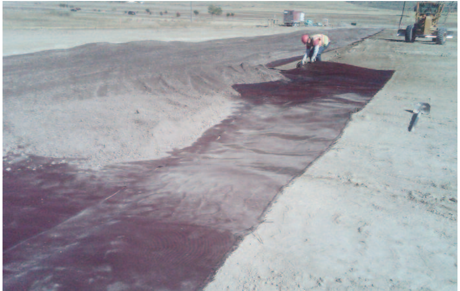
Base material being spread on Mirafi® RS580i.
