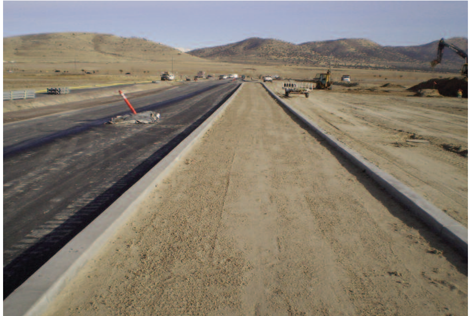
Phased construction - West lanes paved and open to construction traffic.
