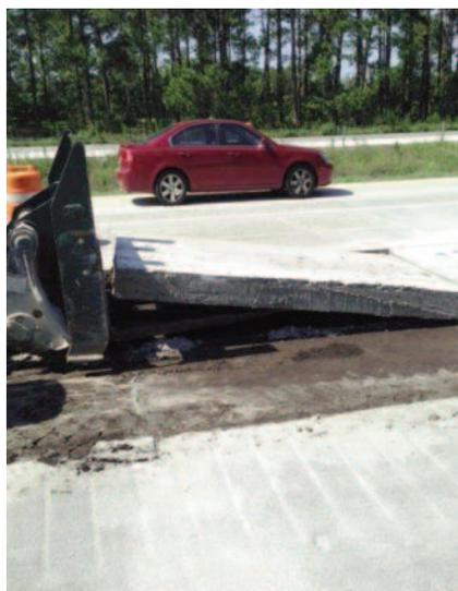
Removal of the existing concrete roadway.
