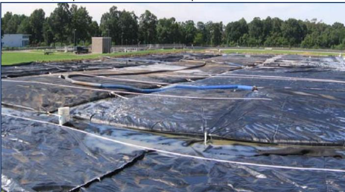
Geotube® units were deployed on Mirafi® NT100-lined dewatering cell.
