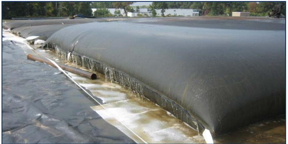
Geotube® Filtration Fabric, (GFF), a 3D drainage media, was placed on the membrane to insure optimum drainage on the bottom of the Geotube® container.
