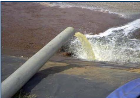
Clean effluent draining directly back into the basin.
