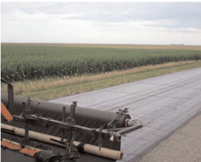
After the asphalt cement was applied to the existing pavement, Mirafi® MPV500 was installed.
