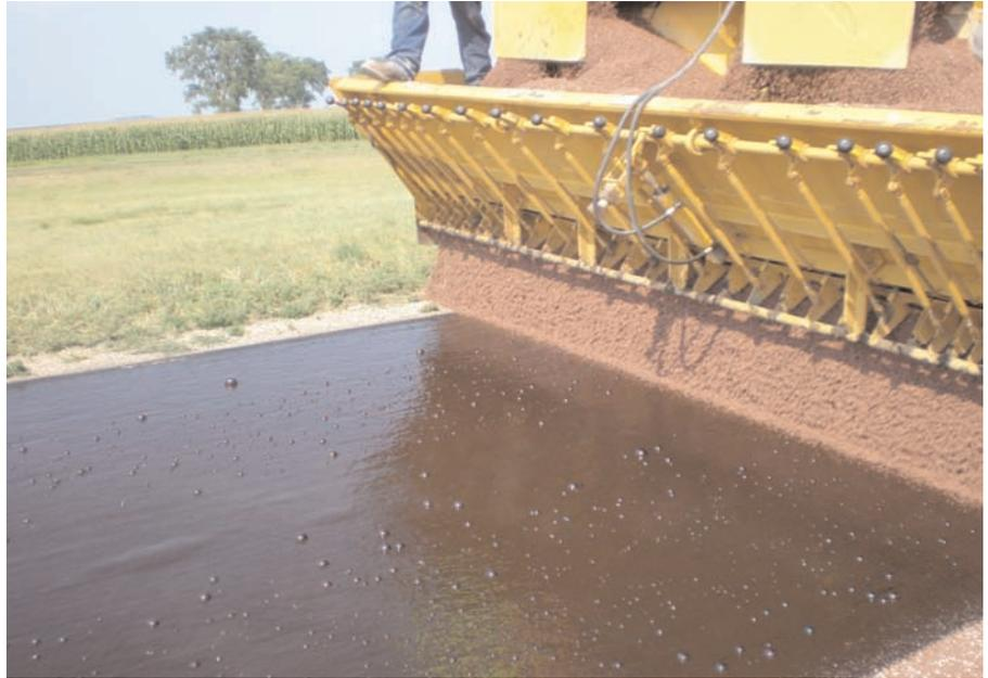
**Above:** The chip seal aggregate was applied using a chip spreader.
