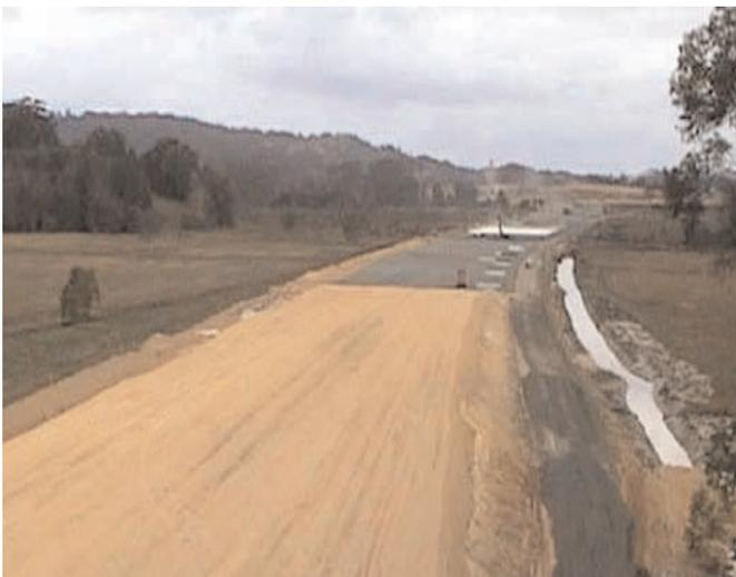
Mirafi® woven polyester was placed on top of the drainage layer to provide reinforcement stability for the embankments.
