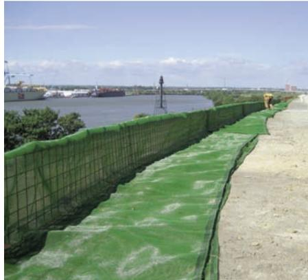
Facing installation showing Miramesh® GR draped over the wire mesh used as form work.
