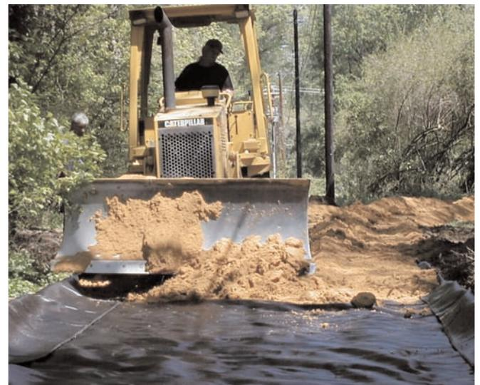
By using a geotextile, costs were minimized by using the existing ground fill.
