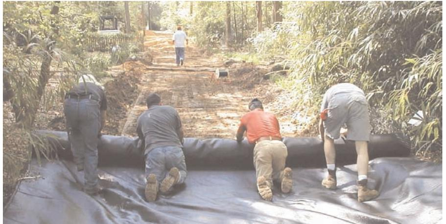
The Mirafi® HP370 permanently stabilized easement supports the heavy water trucks and operational equipment.
