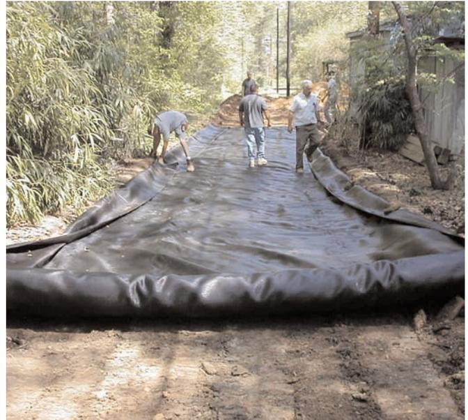
This project required a high strength geotextile due to the weak soils and perched water table.
