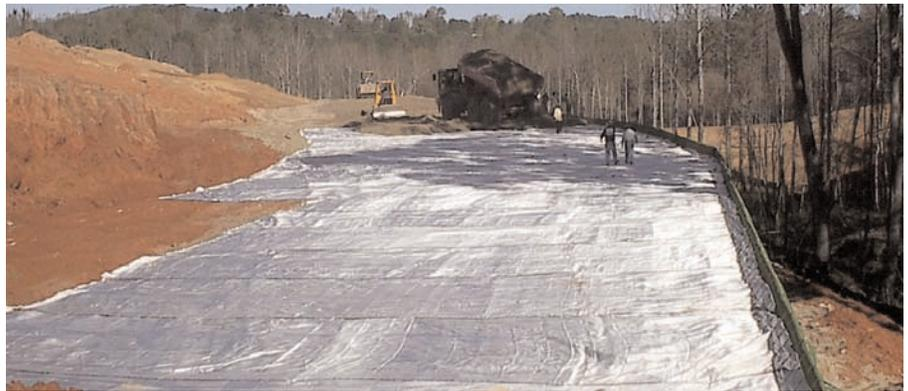
**Above:** The HS400PP and HS800PP high strength geotextiles were embedded between 4.5-6m (15-20ft) in length.
