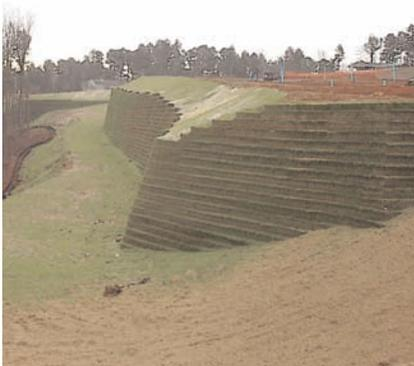
Mirafi® MMESH biaxial geogrid is specifically designed for secondary reinforcement and erosion protection in steepened slopes.
