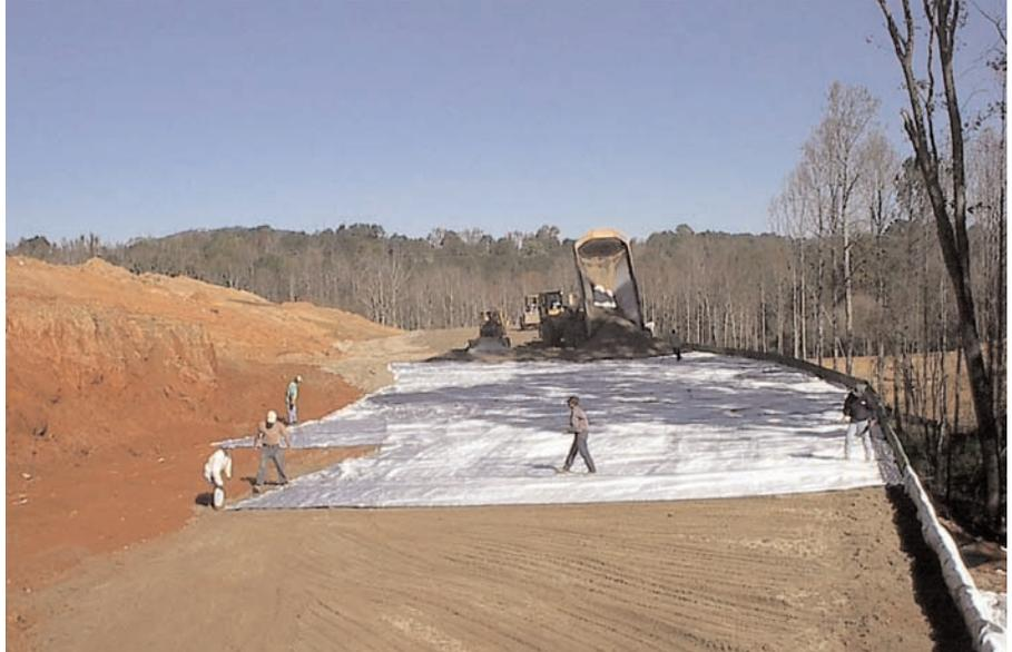
To complete this reinforced slope, 44,733m<sup>2</sup> (53,500yd<sup>2</sup>) of the HS400PP and 48,495m<sup>2</sup> (58,000yd<sup>2</sup>) of the HS800PP were installed as primary reinforcement.
