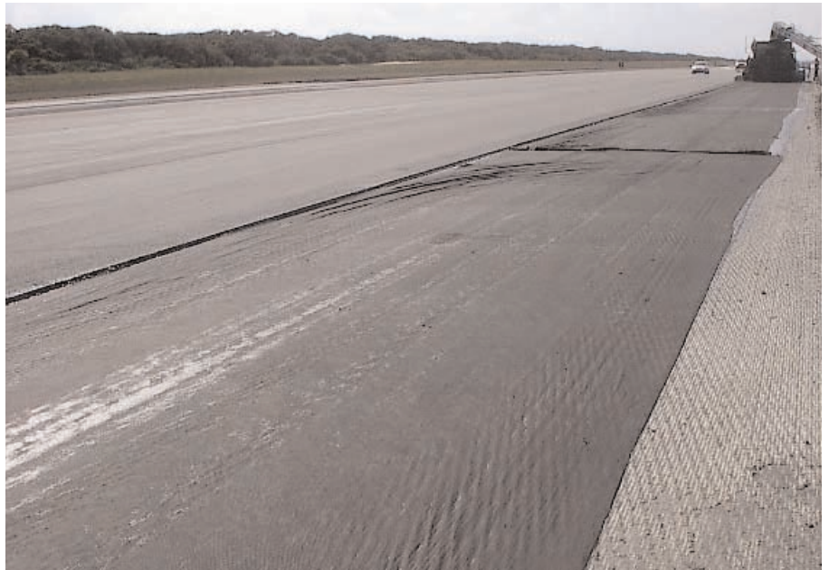
Below: Mirafi® MPV 400 applied with 0.25 gal/sy of tack coat.
