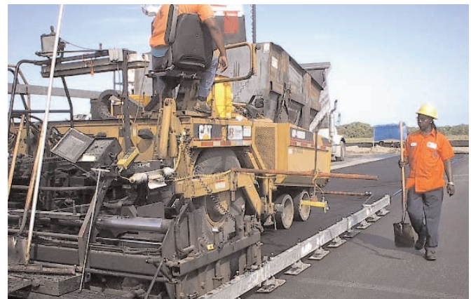
A smooth drummed roller follows the screed machine for proper compaction.
