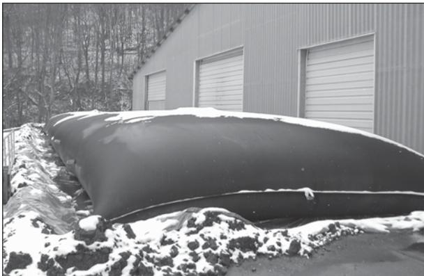
312,000 gallons of heavy sludge were pumped into this Geotube® container. After 45 days, the solids were removed and taken to the landfill.
