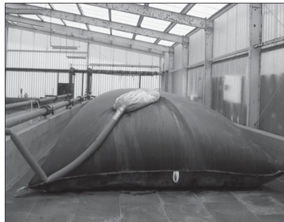
By March 2004, Cambridge WWTP had treated over 900,000 gallons using Geotube® containers.
