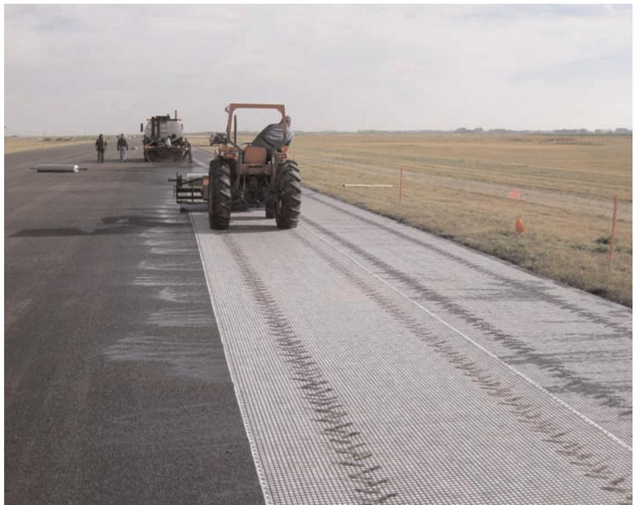
Deploying Mirafi® FG100 over the asphalt levelling course.
