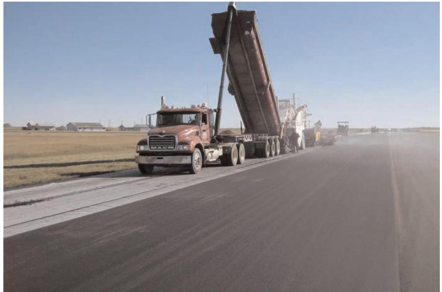
Installing the asphalt overlay on Mirafi® FG100.
