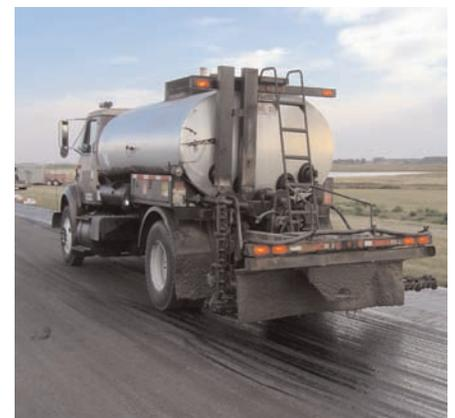
Asphalt emulsion tack coat being applied.
