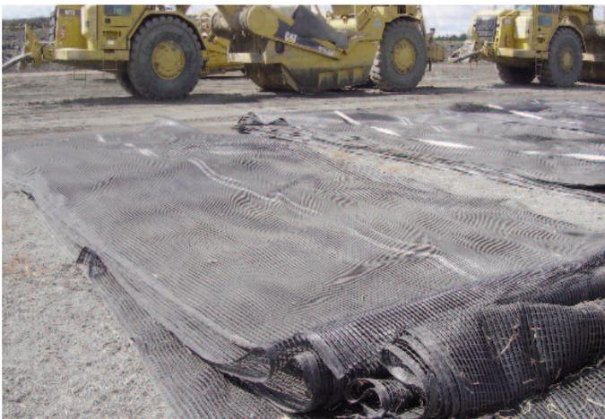
Due to the flexibility and ease of handling of the Miragrid® 8XT, the contractor was able to precut to embedment lengths prior to placement.
