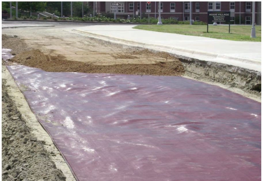
Recycled concrete being placed on Mirafi® RS580i.
