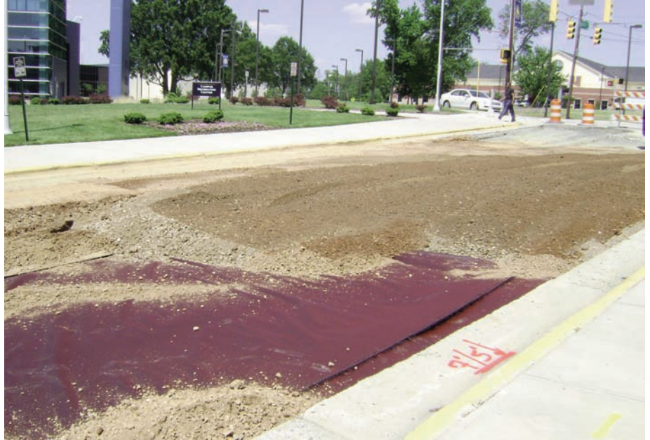
Final aggregate lifts being placed over the material.
