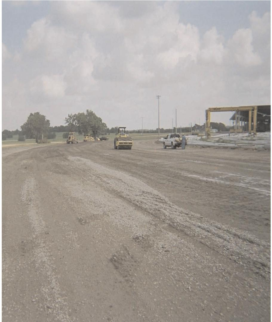
Newly constructed gantry crane wheel path area where Mirafi® HP770 was installed.
