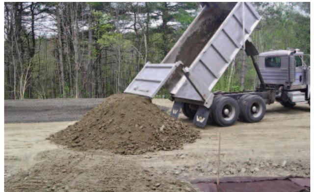
Installation of gravel layer over Mirafi® RS580i.
