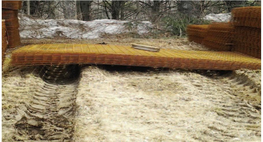
Rutting in the ground's surface from forklift traffic.
