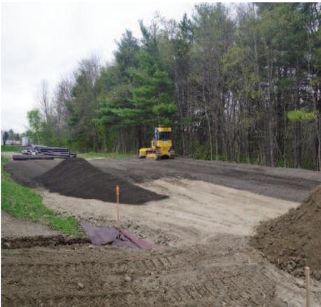
Placing reclaimed asphalt over the compacted gravel.
