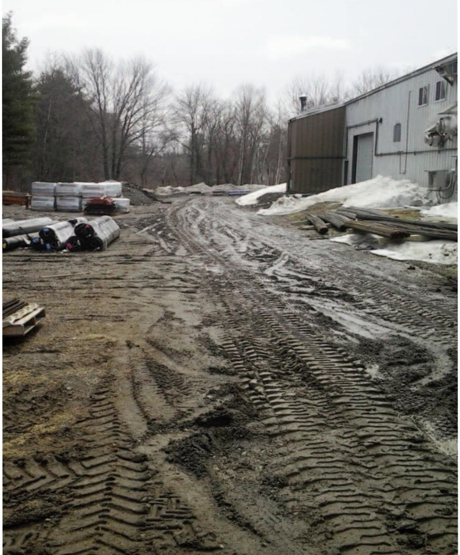
Soft, wet and weak subgrade soils before placement of Mirafi® RS580i.
