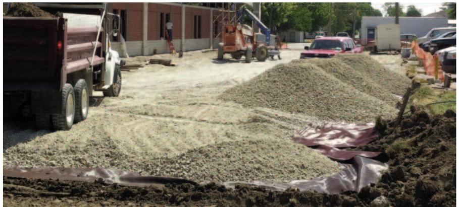
Stabilized site using Mirafi® RS580i geotextile and stone.
