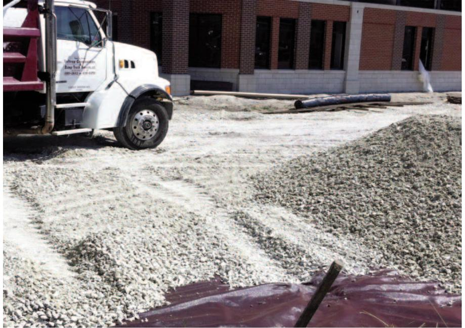
Stabilized site using Mirafi® RS580i geotextile and stone.
