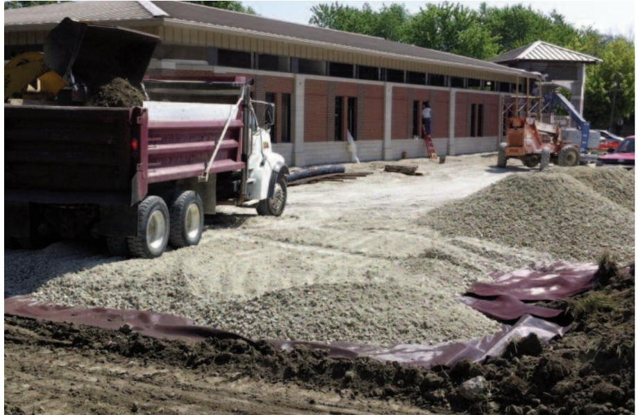
Stabilized site using Mirafi® RS580i geotextile and stone.
