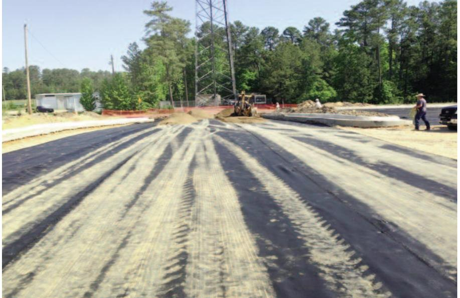
Installation of base course aggregate over Mirafi® HP570 geotextile.
