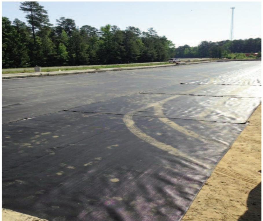
Installation of Mirafi® HP570 geotextile.
