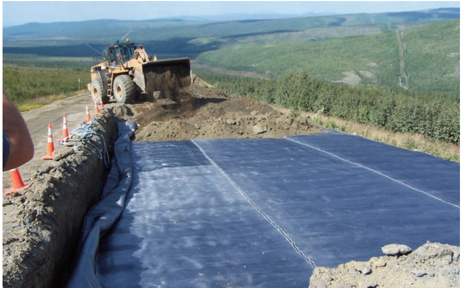
Installation of Mirafi® H 2 Ri on the Beaver Slide area.
