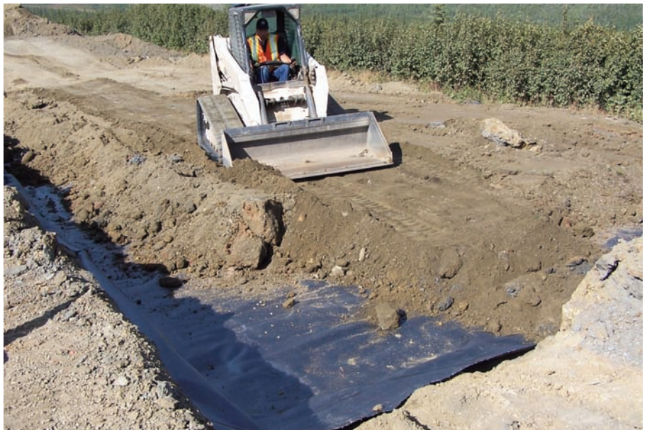
Spreading of base course over Mirafi® H 2 Ri geosynthetic.
